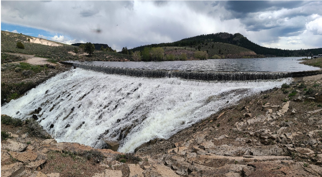
Caption: Downstream slope of dam while reservoir is spilling.
