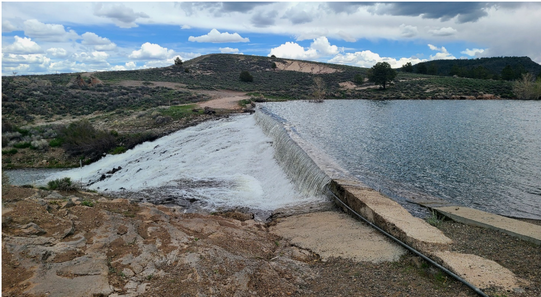
Caption: Dam crest while reservoir is spilling.
