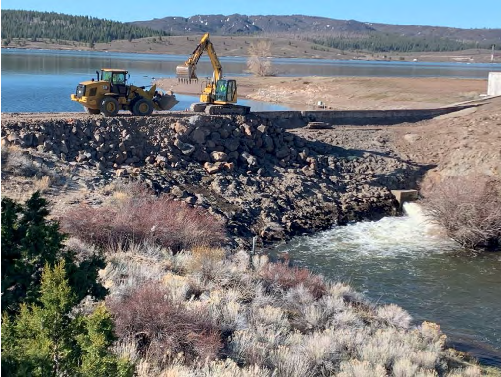
Rockfill berm being removed
