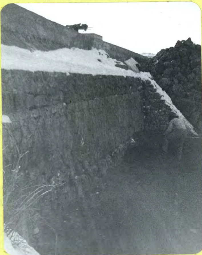
#7 Placement of natural fill material over imported fill material. (Approx. 18" in depth) east side of culvert extension.
