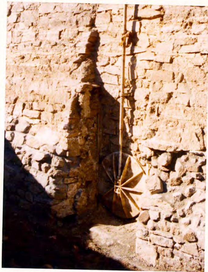
#1 Nov. 1975. Panguitch Dam, 48" dia. slide gate. Invert to crest of dam 24' - 2".
