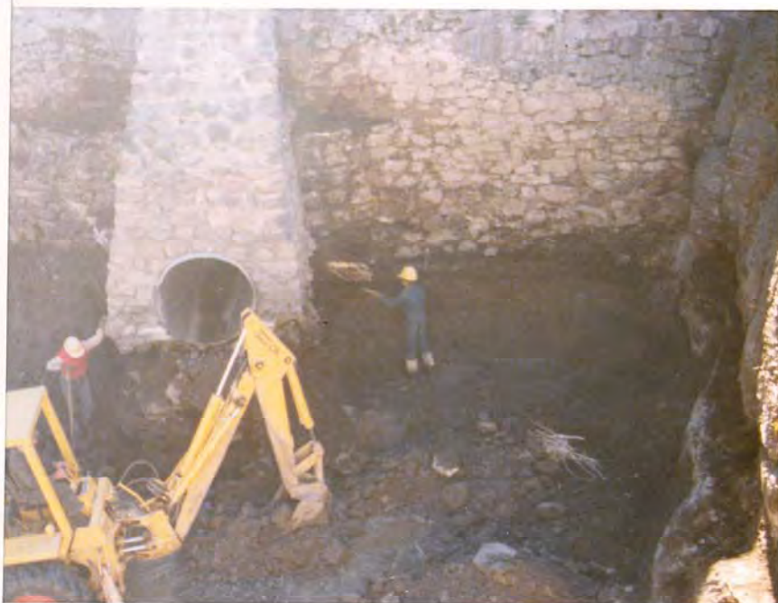
#4 Panguitch Lake Dam. Nov. 1975. Removal of existing material; downstream face.
