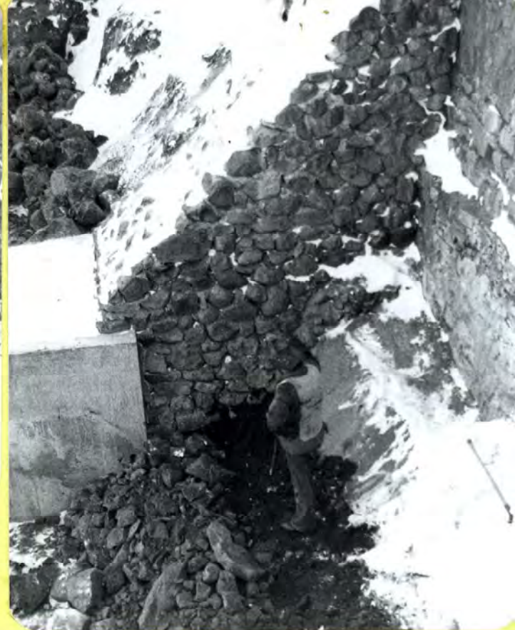
#1 and #2 Placement of fill material against downstream face of dam. Imported fill is light and natural fill is dark.
