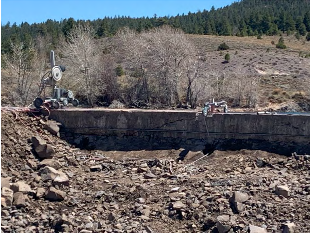
Wire saw set up for vertical cut at Sta 1+04
