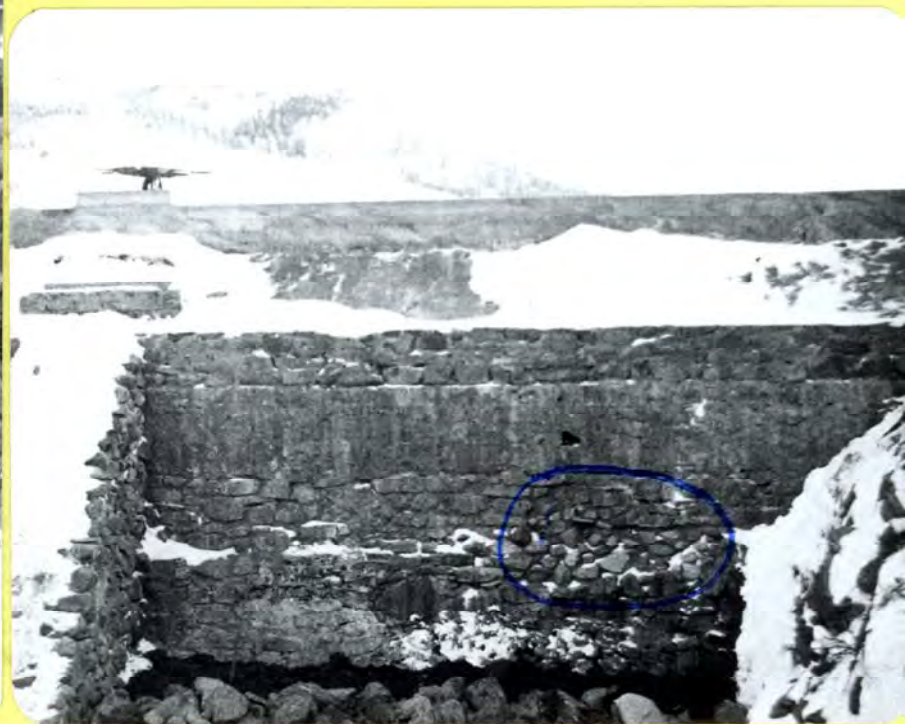
#4 REPAIRED Required downstream face cavity was about 6 feet below outside edge and on the right side near the west
