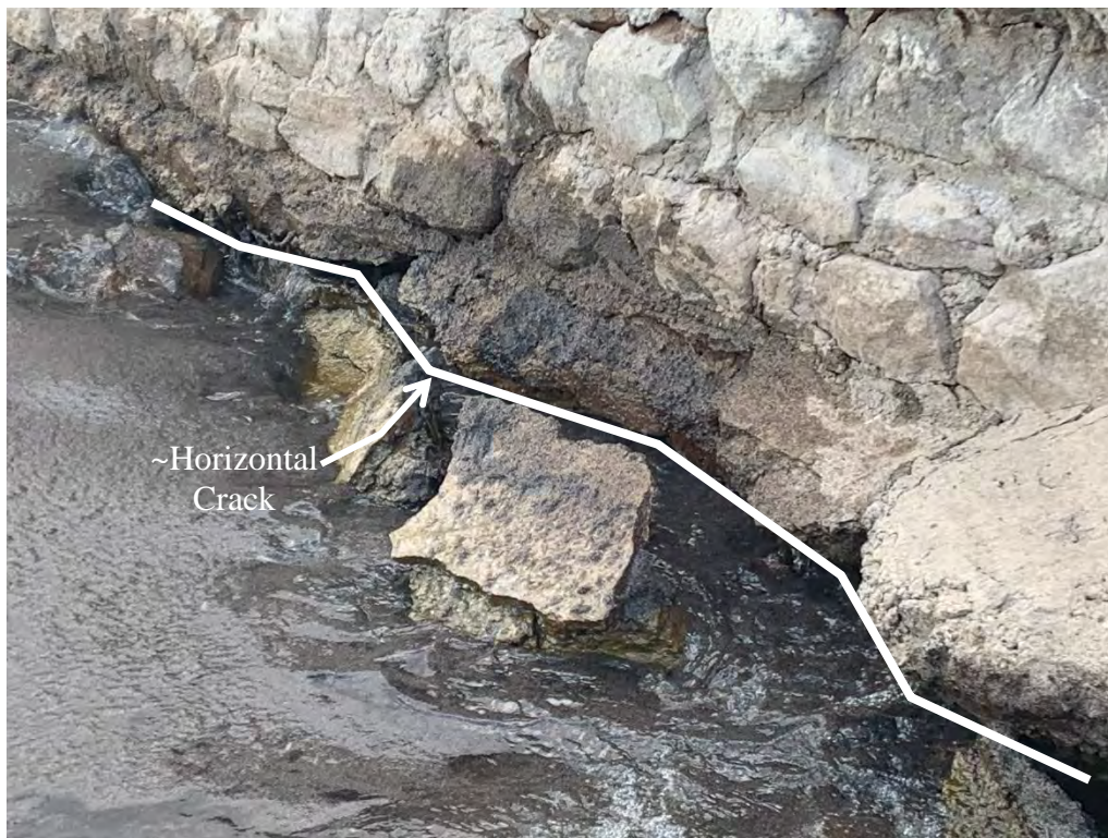
Upstream dam face, near right abutment
