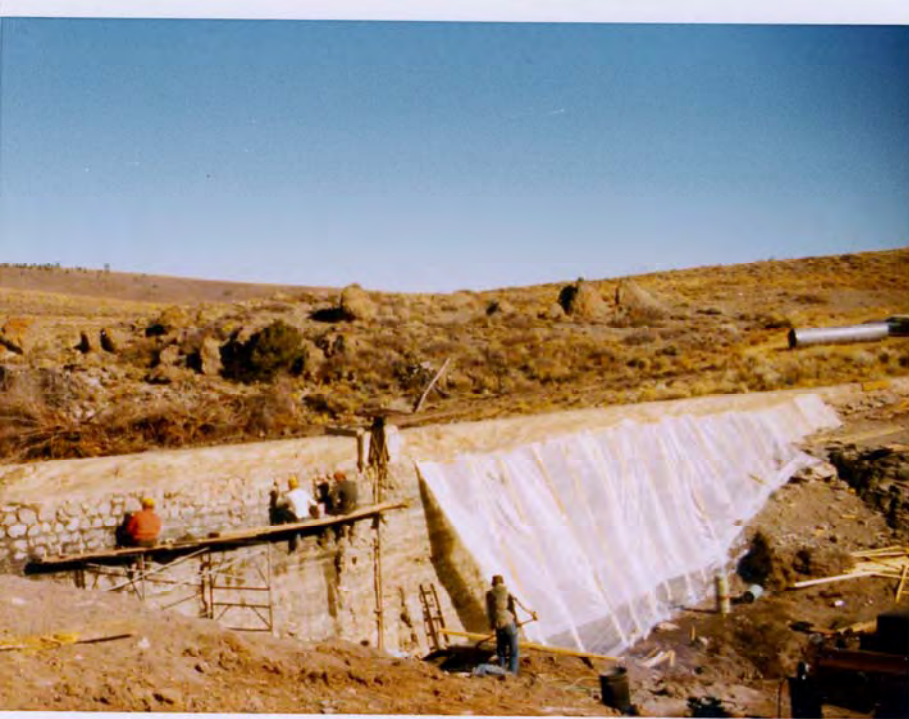
6 Nov. 1975. Panguitch Dam. Upstream mortar repair in progress.
