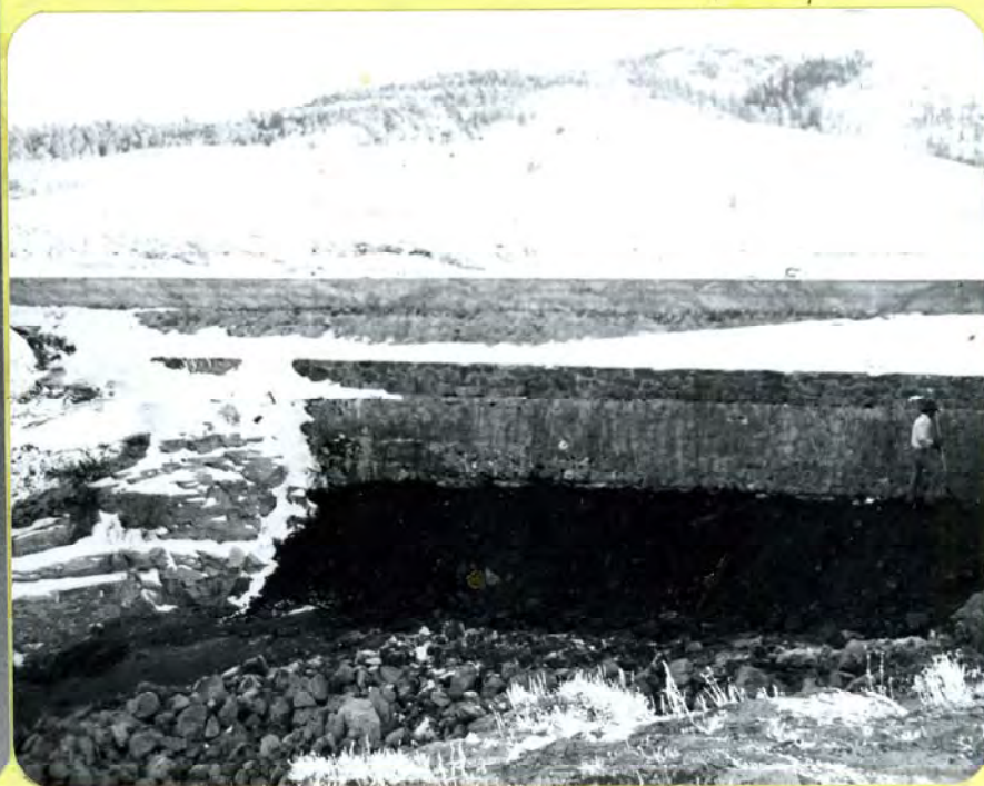
#8 Finished placement of natural fill material against and over imported fill on downstream face of Panguitch Lake Dam.
