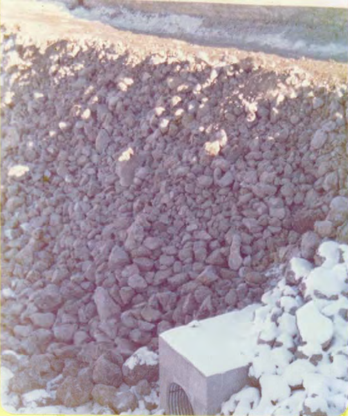
#1 Rockfill placement as completed but prior to final shaping by D-7 Cat.
