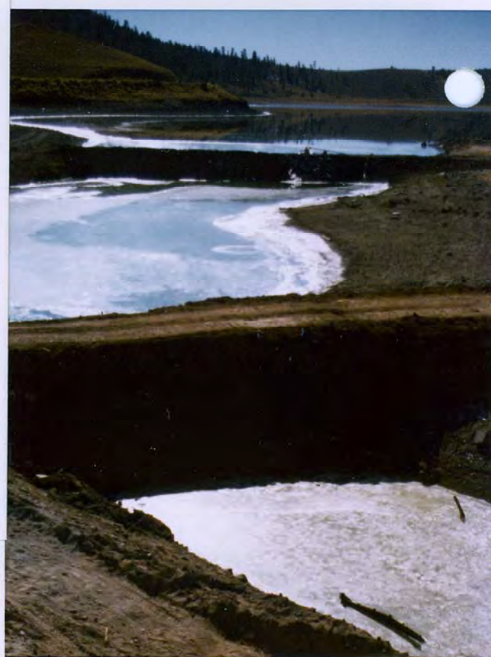
#7 Nov. 1975. Panguitch Dam. View south showing two coffer dams with pumping equipment.
