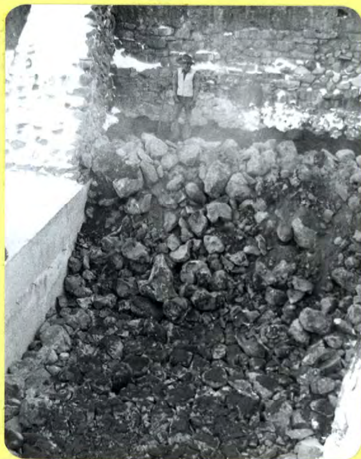
#3 Natural fill brought up and over imported fill. Rock fill started on the west side of the dam.
