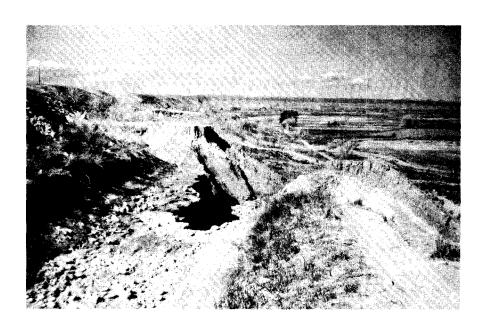
Figure 13.— View looking west of break of April 23, 1972, in Pleasant Valley Canal, showing chute cut in slumped beds of Uinta Formation. Note abundance of vegetation along bluff below canal in distance.
