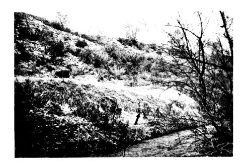
Figure 9.—Landslip between upper and lower Rocky Point Canals at location U(C-3-4)32aba. The tongue (arrow) of the slip is covered with saltgrass (Distichlis stricta) and has moved from left to right (in photograph), with edge of tongue on lower canal.
